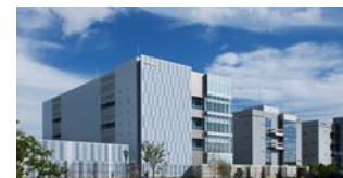
Okayama Data Center
