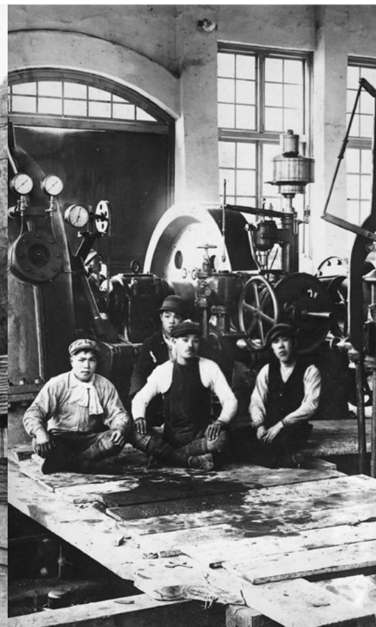
The power station at the Hitachi mine (1916)
